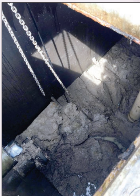
Holding tank restricted by paper build-up.
